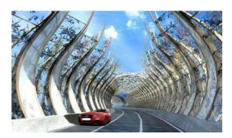
Photovoltiac noise barrier, A13 motorway, Switzerland (Fanzun, Architects and Engineers). The world's first photovoltaic noise barrier, and recently renewed with three times original output. The 800m2 barriers provides power for 92 homes
